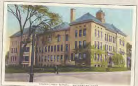
A postcard dated 1916 shows Crosby High School on East Main Street in Waterbury, one year before an addition would begin being built on site.
